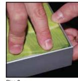
Repeat Step 1 for opposite corner C, then insert corner B, followed by corner D. to complete the installation of the corners
